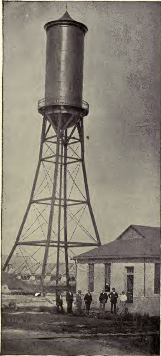
TOWER AND TANK, WEST TAMPA, FLA.
